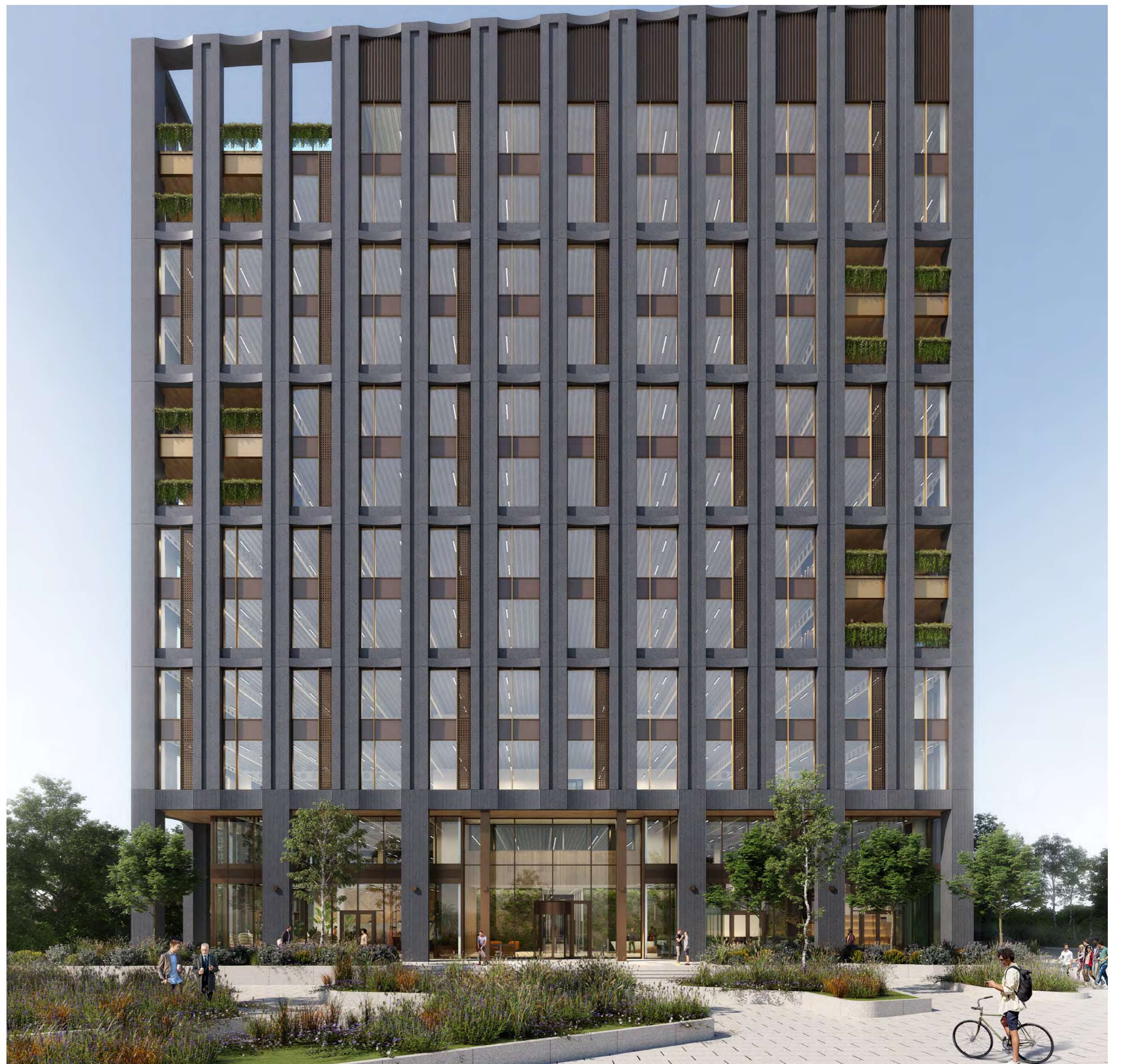
View of southern elevation
