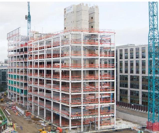
Structural steelwork is almost complete on building 11 and building 12 has also progressed well. We have started the metal decking to building 12 which is also progressing well.
